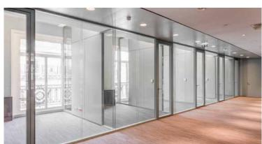
with aluminium profiles. An almost invisible transparant profile makes a nearly seamless junction between the different glass panels.
